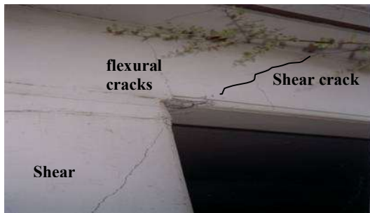
Fig. 1. Damage of T-Beam at the joint with the nearby column (6 th story building, Aharnes, Athens earthquake 1995) [4].
